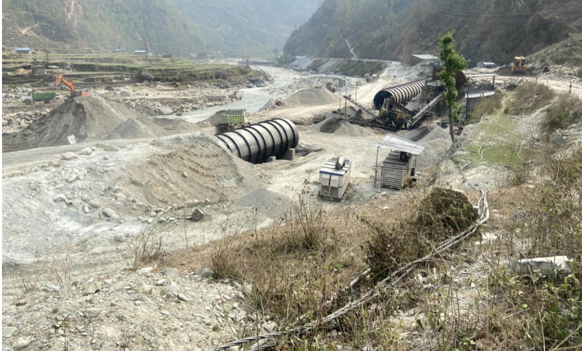
Figure 11: Headrace pipe alignment
