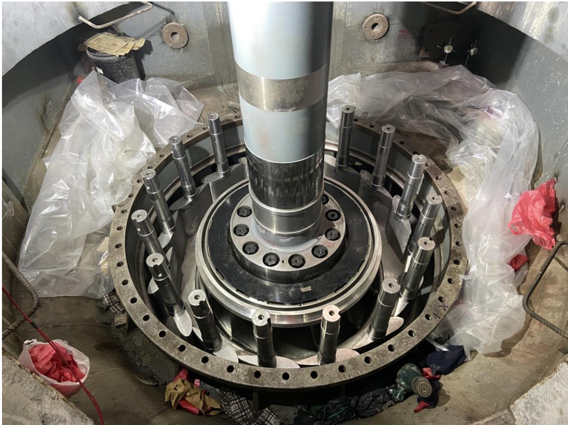
Figure 13: Runner-shaft assembly lowered inside the unit 2 pit
