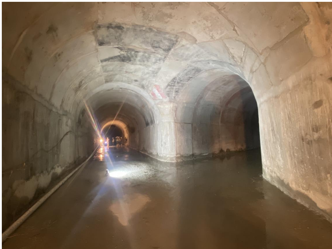
Figure 4: Headrace tunnel (left side) and connecting tunnel to surge shaft (right side)
