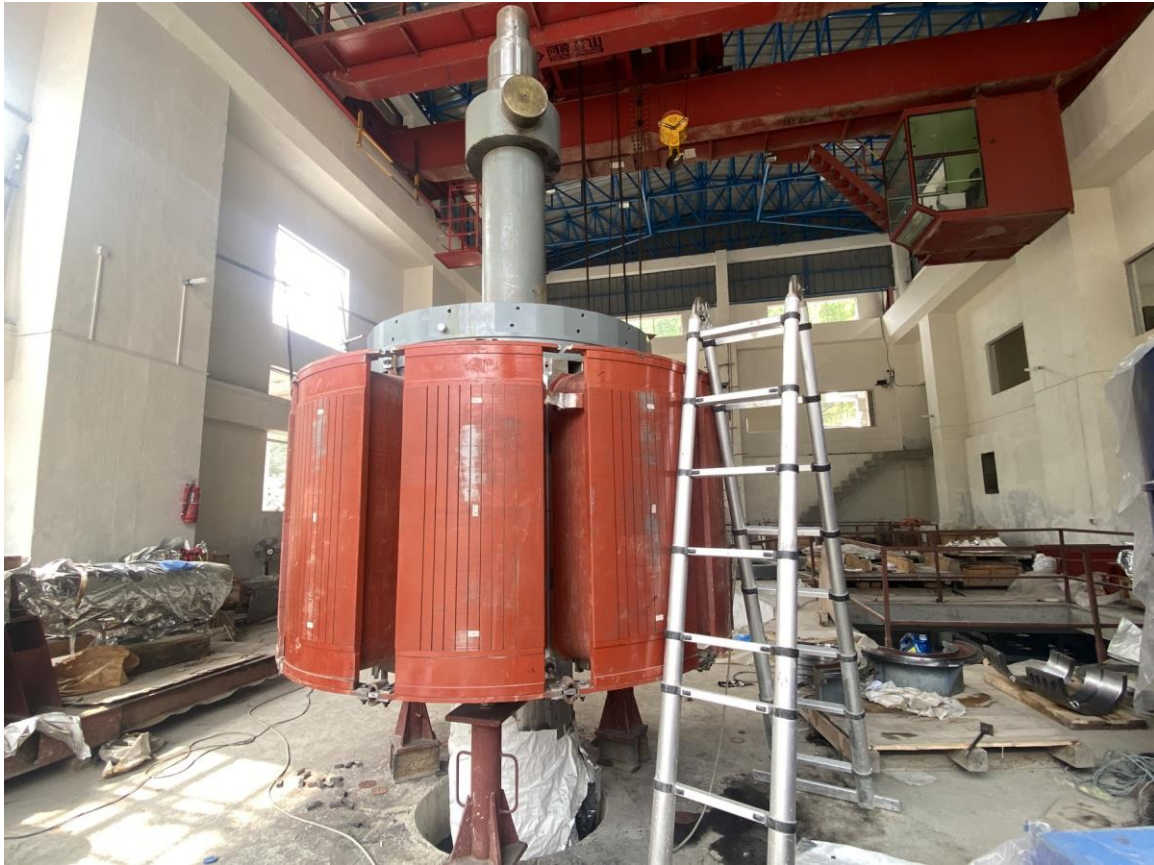
Figure 14: Rotor-pole assembly for unit 2
