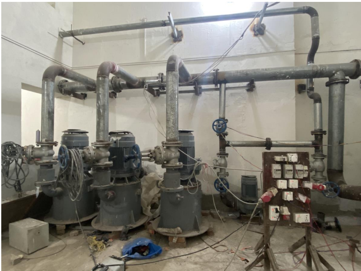
Figure 15: Installation of cooling water pipeline for unit 2
