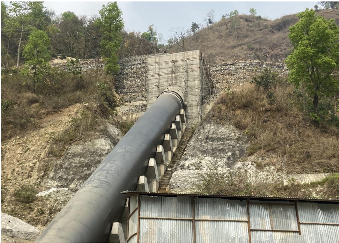
Figure 8: Geo-grid structure at either sides of anchor block VB02
