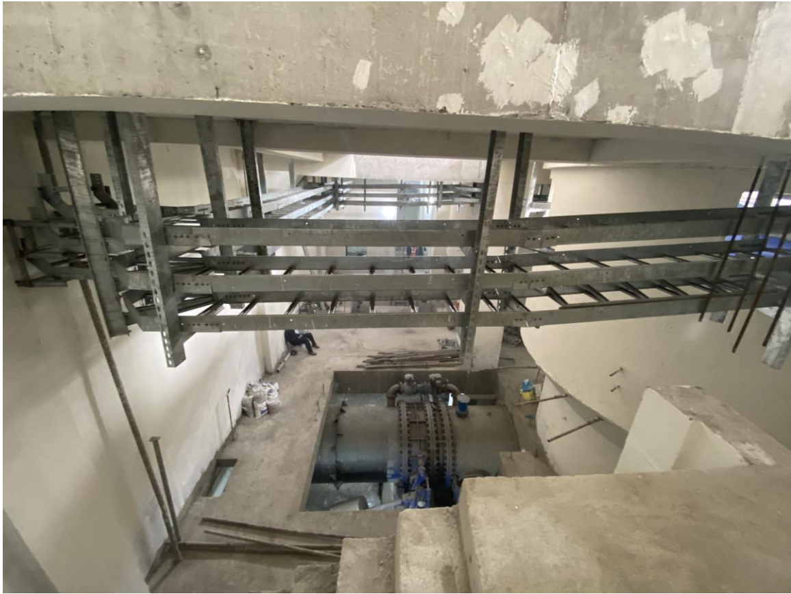
Figure 24: Cable tray installation at powerhouse
