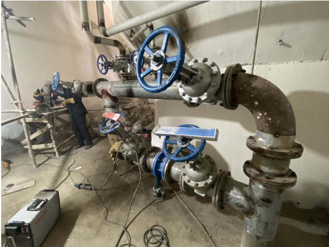
Figure 26: Cooling pipe installation works at Unit 1
