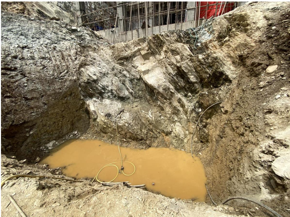
Figure 23: Excavation of penstock anchor block VB01
