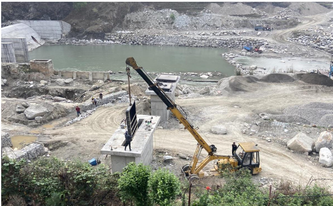
Figure 12: Installation of settling basin inlet gate leaf
