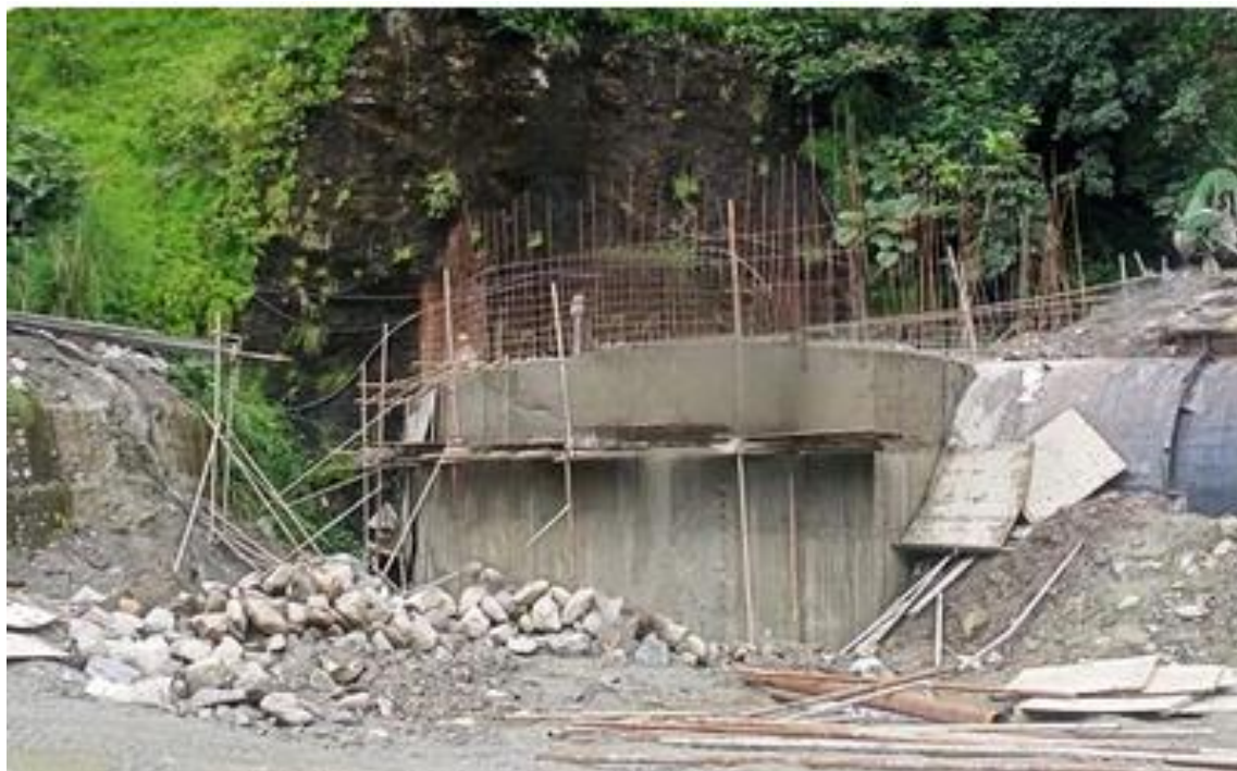
Figure 3: Plum concrete at the main inlet portal anchor block
