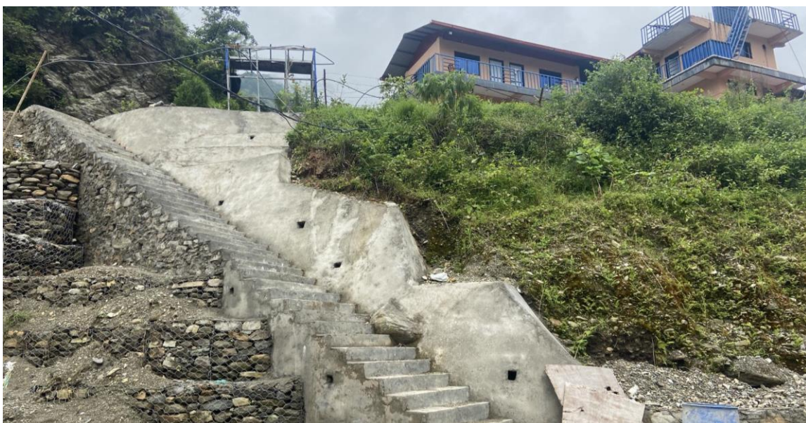
Figure 2: Construction of stairs from settling basin to Headworks staff quarter
