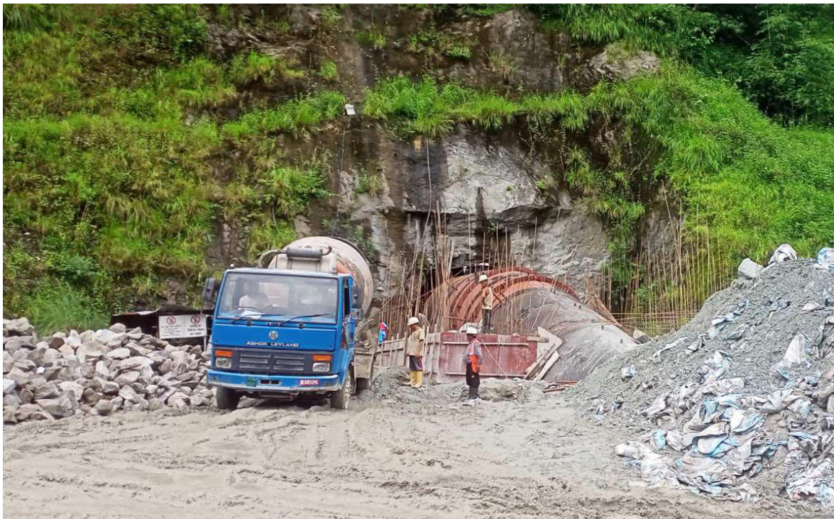
Figure 29: Plum concreting at Seti outlet using Transit Mixer
