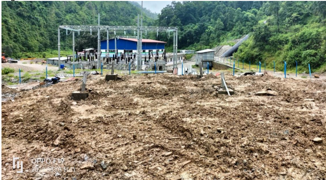
Figure 15: Foundation backfilling at AP00
