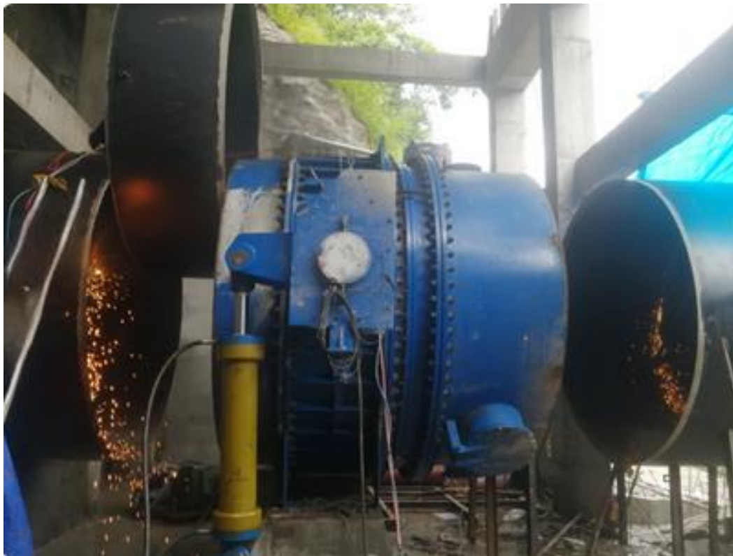
Figure 23: Welding works at PPV house
