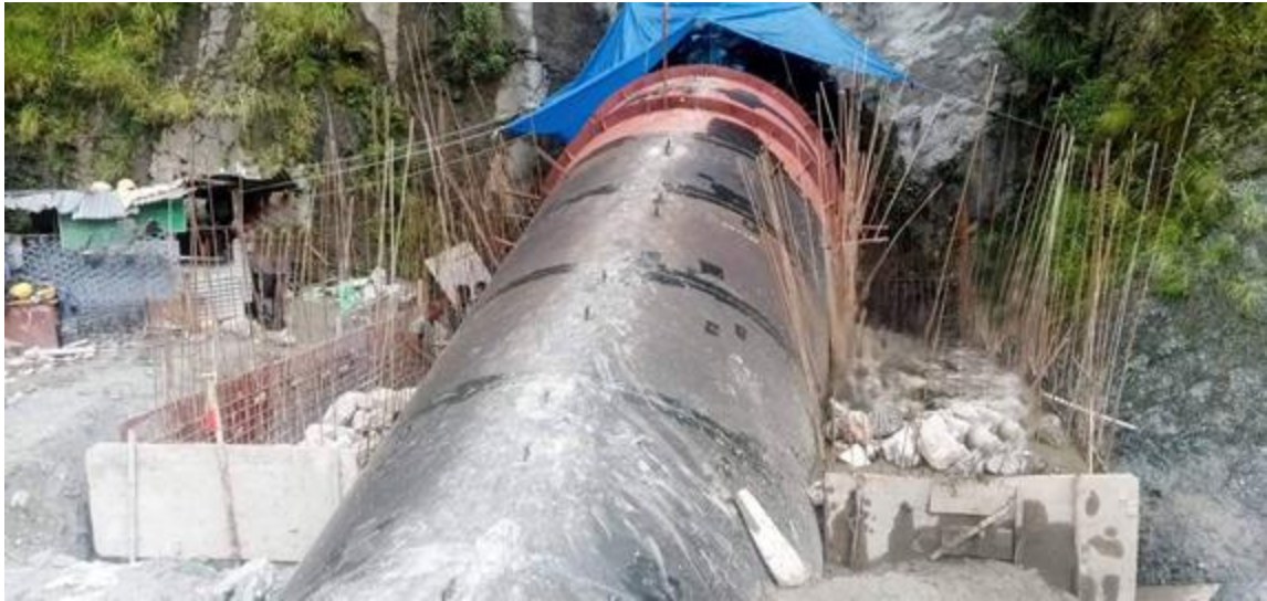
Figure 4: Plum concrete works at Seti outlet anchor block
