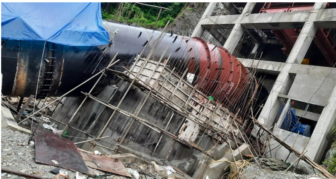
Figure 9: Penstock pipe bend (VB01)
