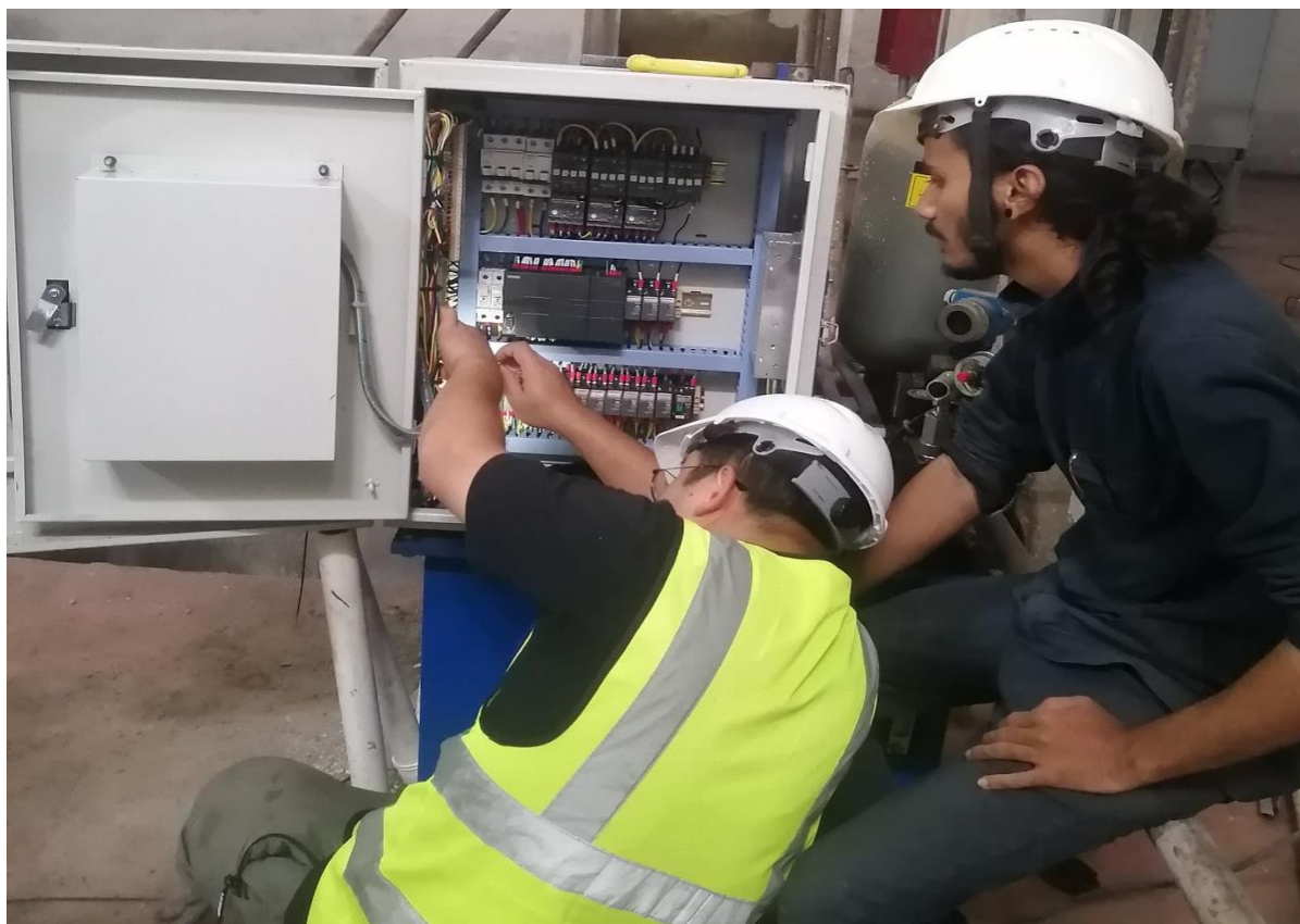
Figure 11: MIV control panel installation
