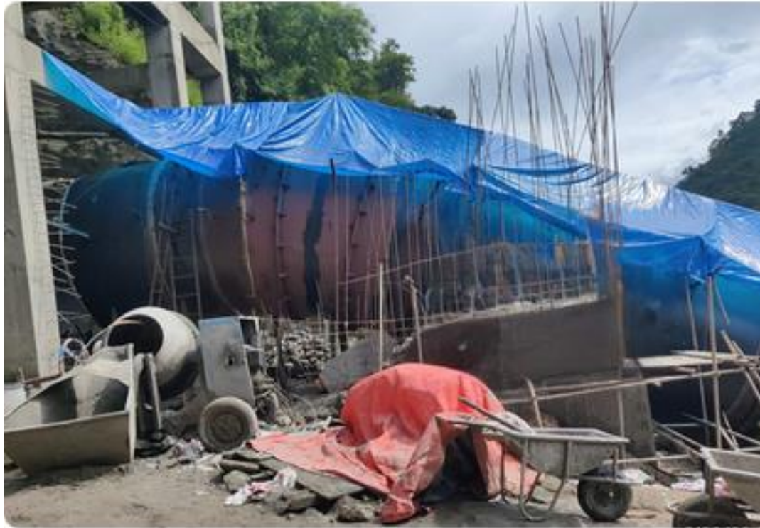
Figure 22: Plum concrete works at anchor block VB01 of penstock
