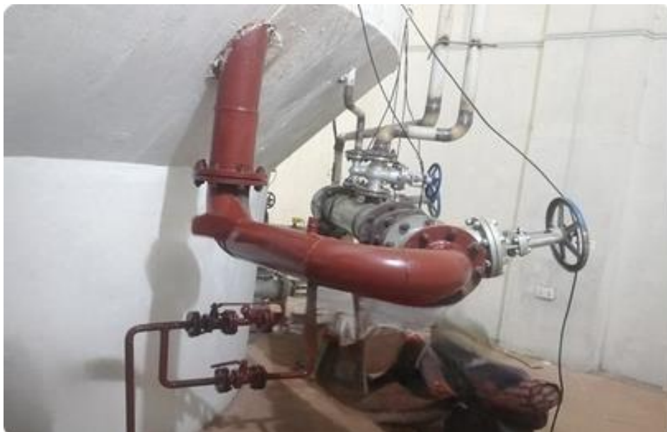
Figure 10: Red Oxide painting on cooling pipeline system
