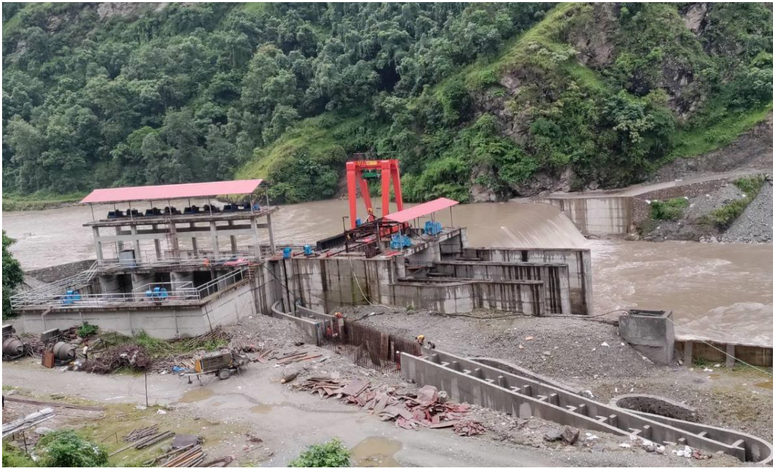
Figure 20: View of weir, undersluice and intake
