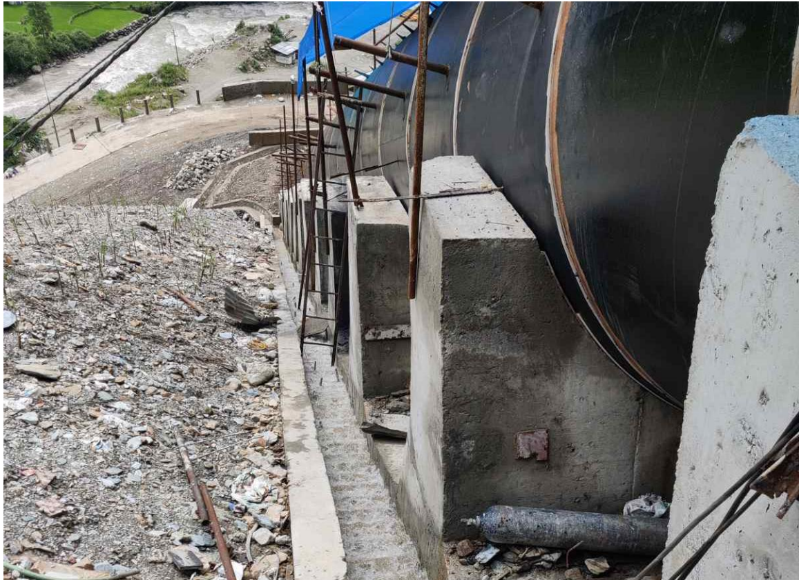
Figure 6: Side drainage at the penstock alignment
