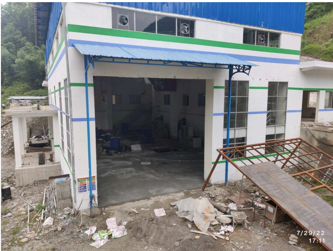
Figure 25: Floor finishing at machine hall level
