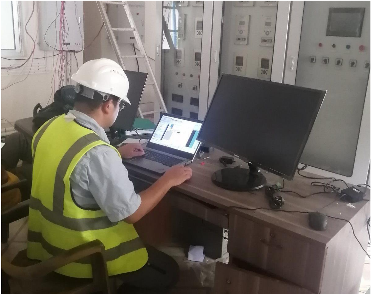
Figure 13: PLC and SCADA system testing at control room
