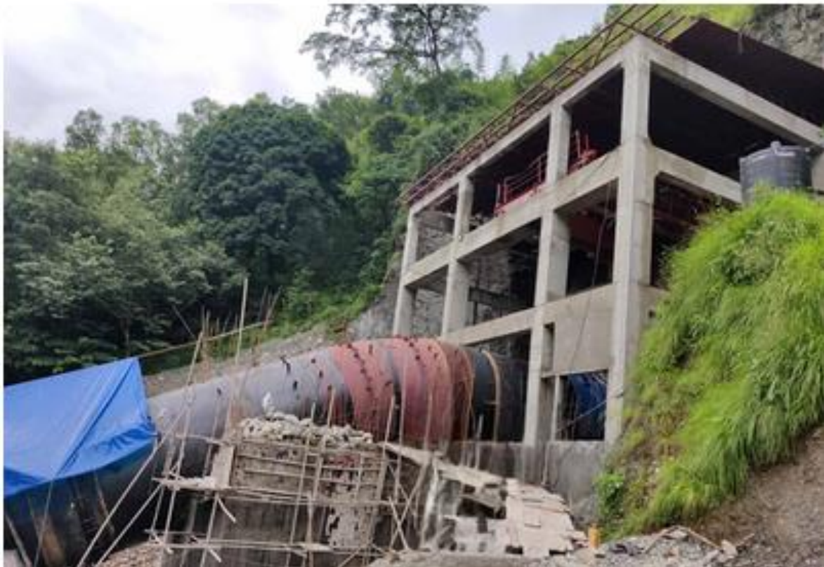
Figure 5: Construction of anchor block VB01 of penstock and PPV house roofing
