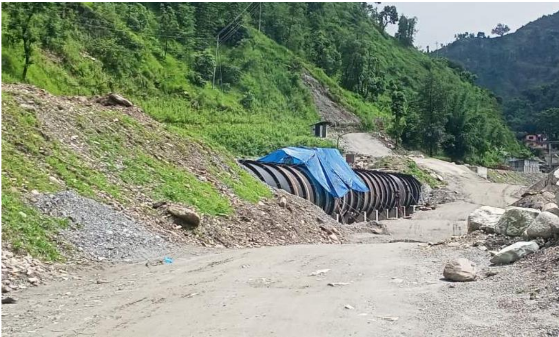
Figure 8: Headrace pipe
