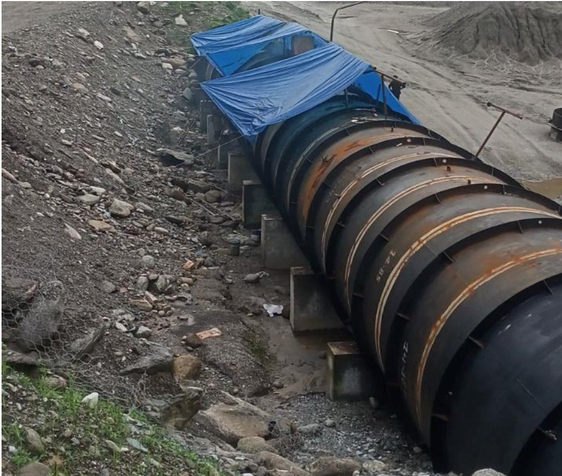
Figure 24: Welding at headrace pipe
