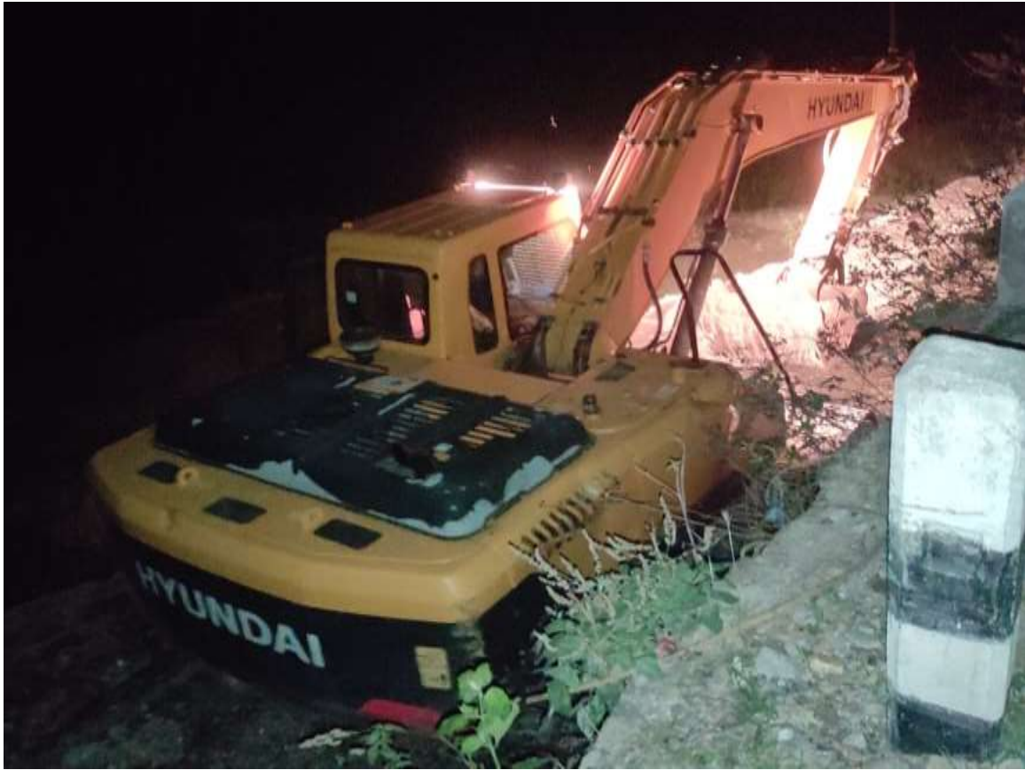
Figure 30: Excavation of tower foundation at AP 63
