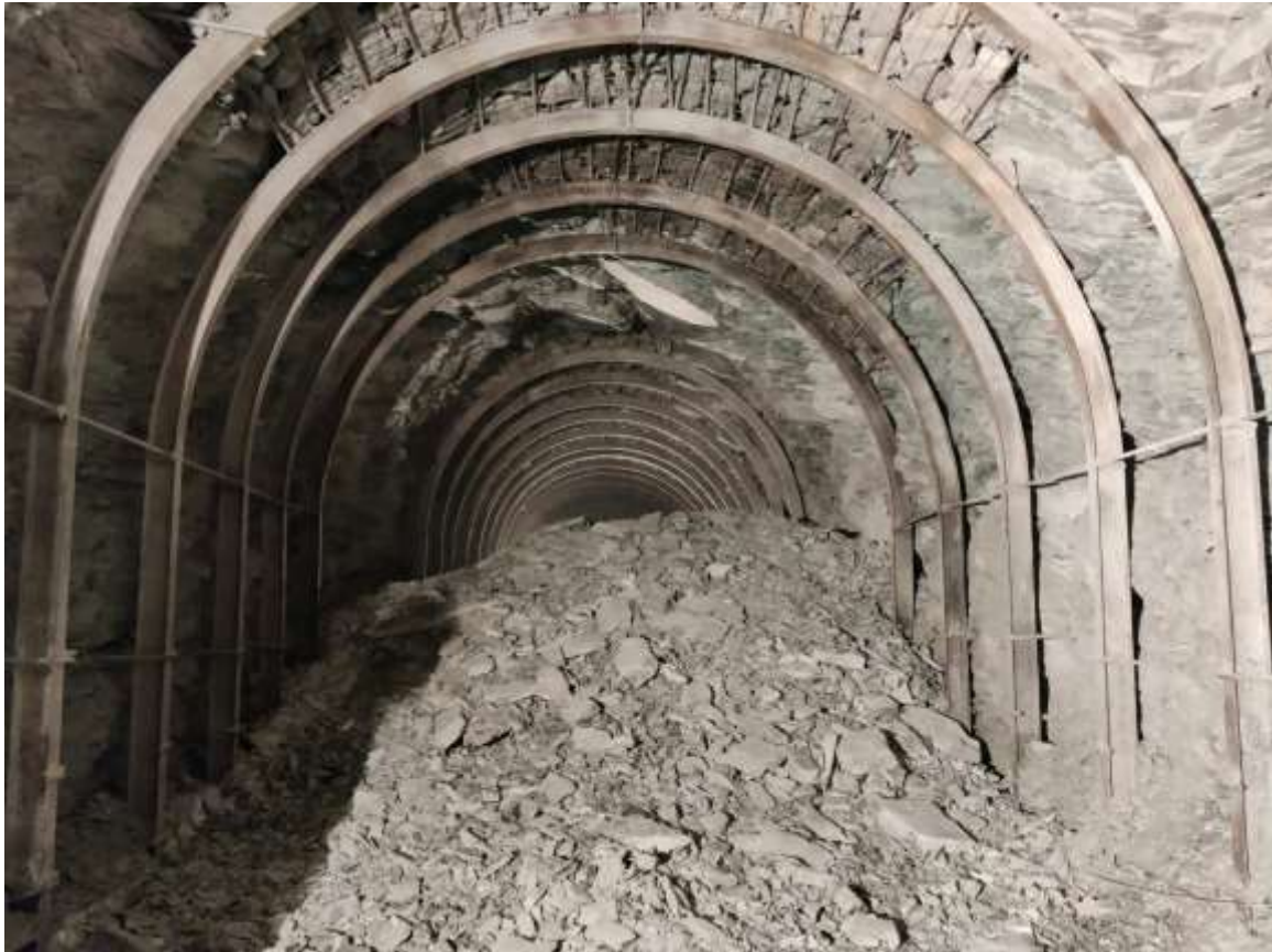
Figure 24: Breakthrough of tunnel stretch between Face 1 and Face 2
