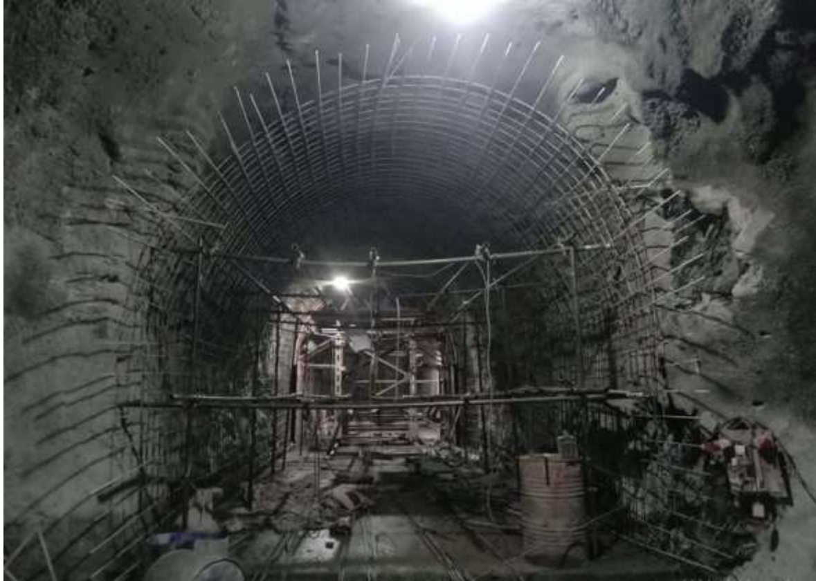
Figure 6: Reinforcement installation for full concrete lining at Face 5
