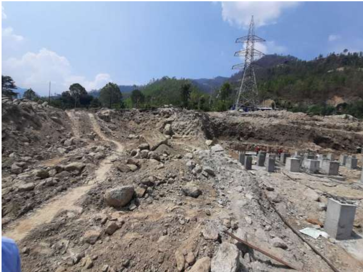
Figure 17: Excavation for LLHP bay at New Khimti Substation
