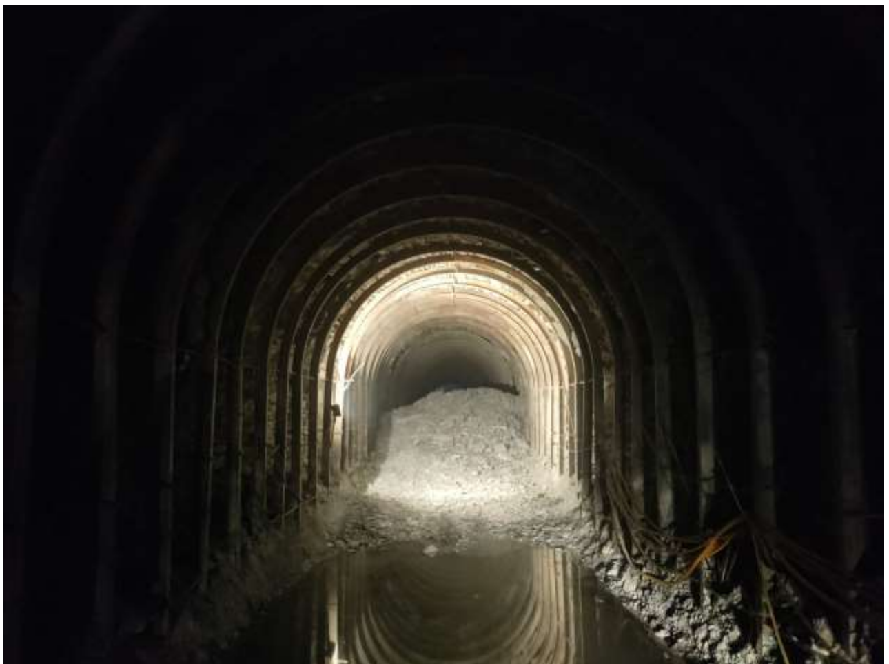
Figure 5: Breakthrough of tunnel stretch between Face 01 and Face 02.
