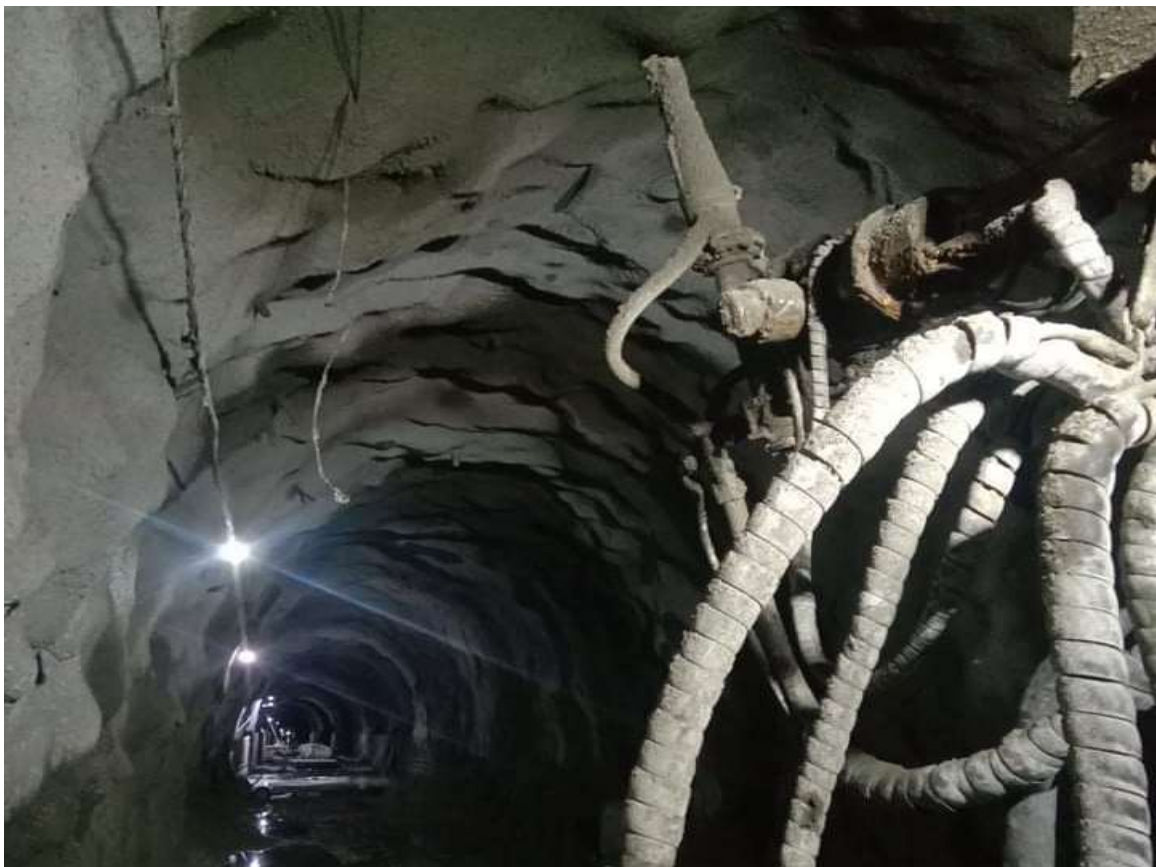
Figure 25: Spraying of shotcrete inside the tunnel (Face 5)
