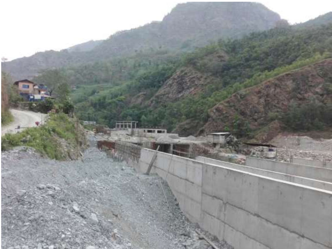
Figure 2: Hillside walls of Settling basin panel 4, 5,6
