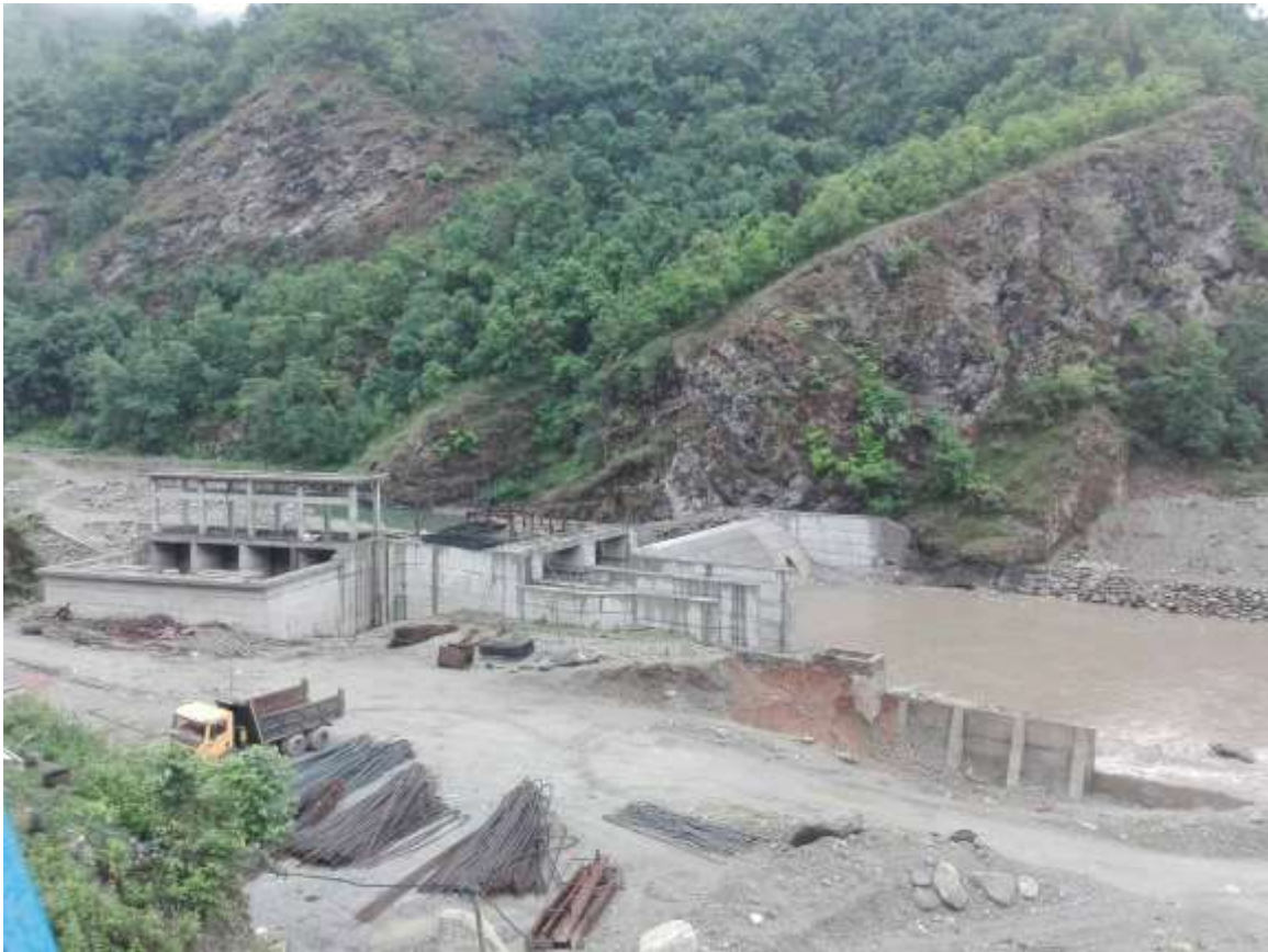
Figure 22: View of weir, intake and undersluice including retaining wall at left bank
