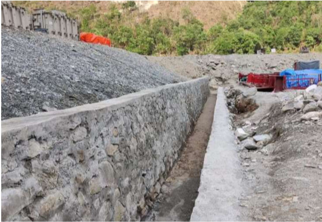
Figure 12: Drainage works at switchyard boundary
