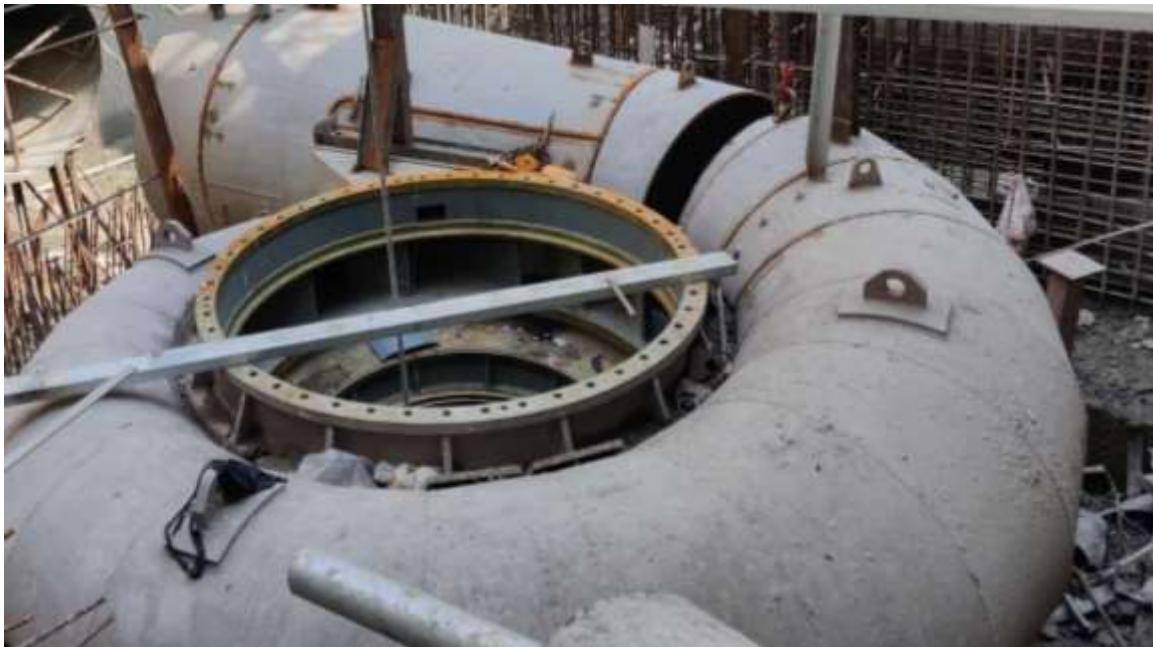
Figure 15: Spiral case installation in Bay 01
