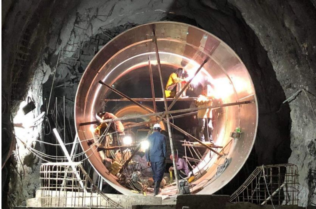
Figure 8: Pipe installation at the Seti Outlet portal side
