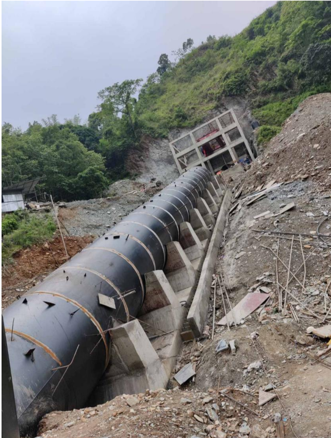
Figure 5: View of the penstock pipe saddle supports and PPV house
