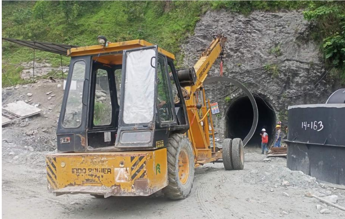
Figure 20: Transport of pipe inside main inlet tunnel using hydraulic crane
