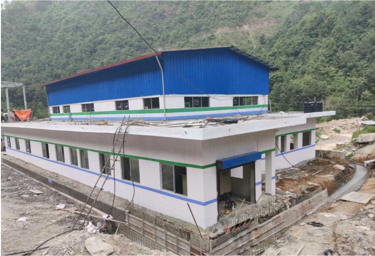
Figure 6: Surface drainage and painting works ongoing in the powerhouse
