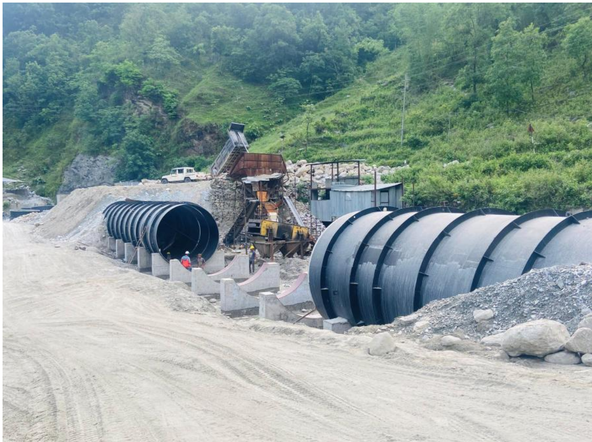
Figure 3: Construction of headrace pipe saddle supports in crusher area
