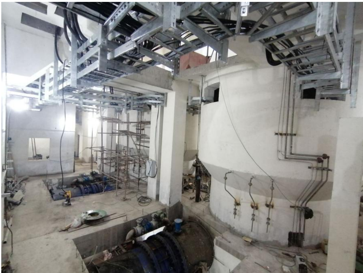
Figure 11: Cable tray and cooling pipeline of machine unit 2
