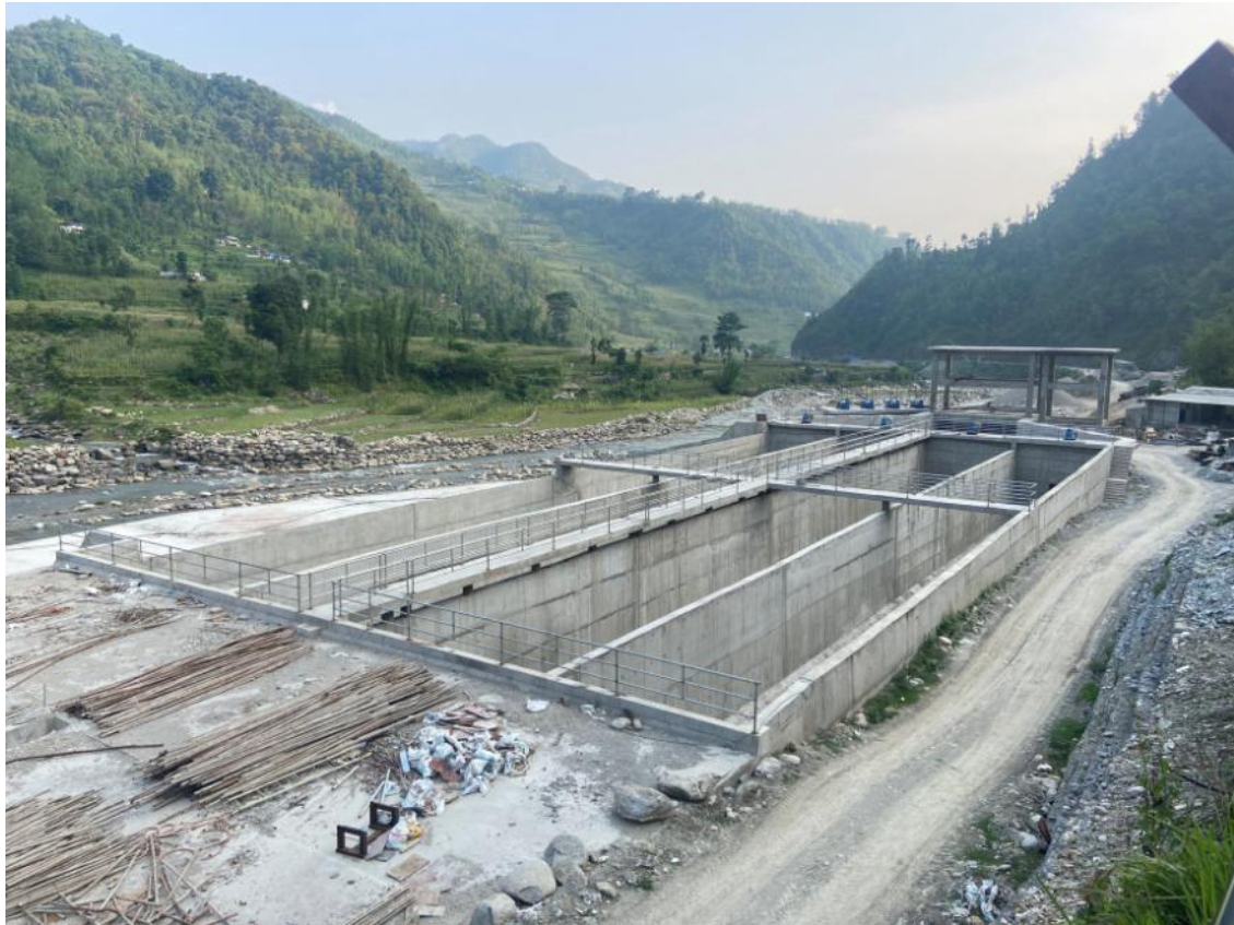
Figure 18: View of settling basin
