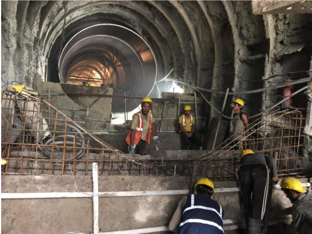
Figure 4: Saddle support construction at the main inlet portal side
