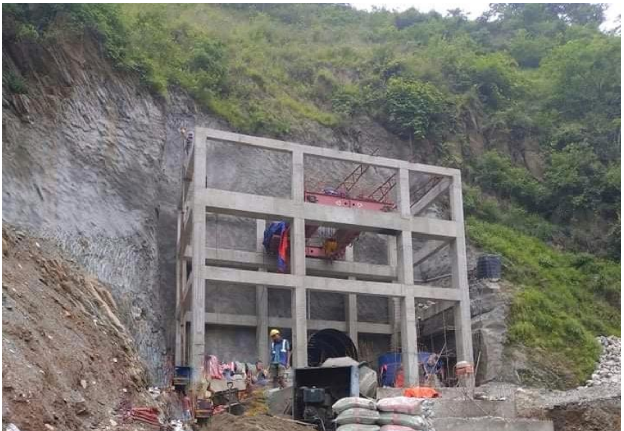
Figure 7: Roof truss installation initiated in the PPV house
