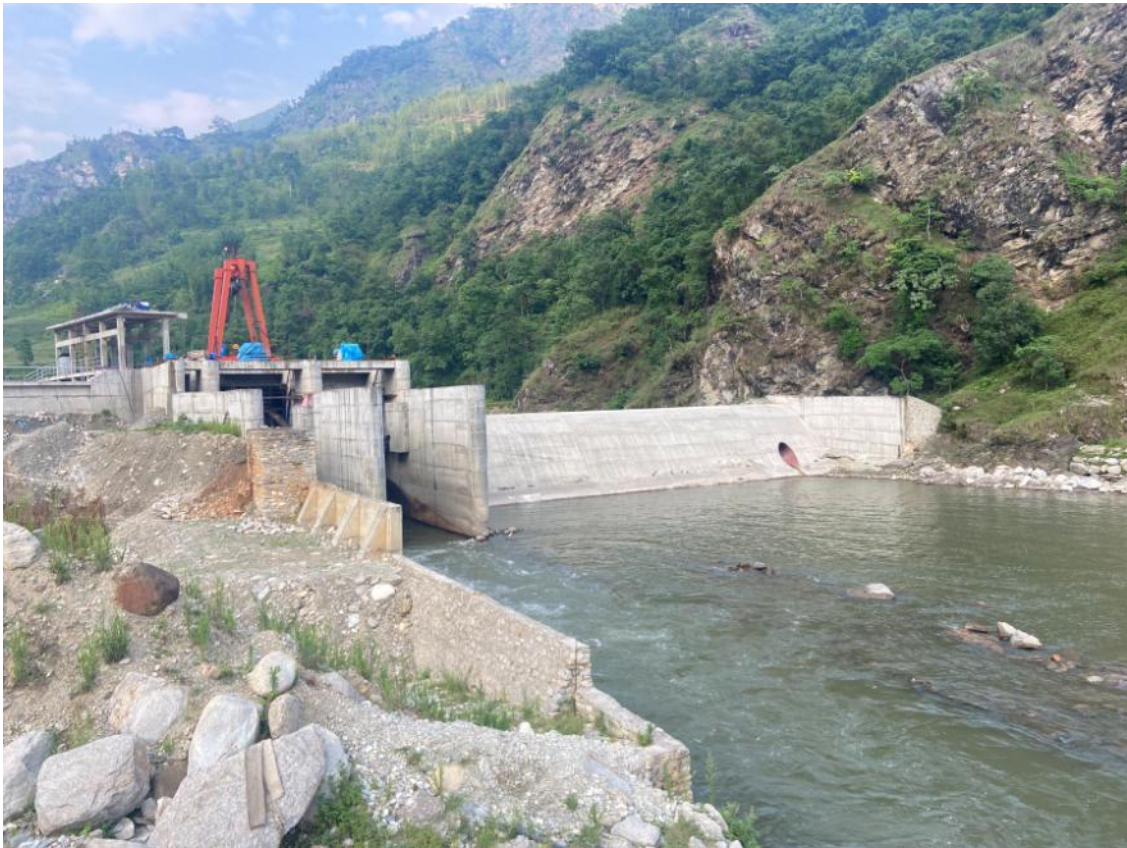
Figure 16: View of weir and undersluice from downstream side
