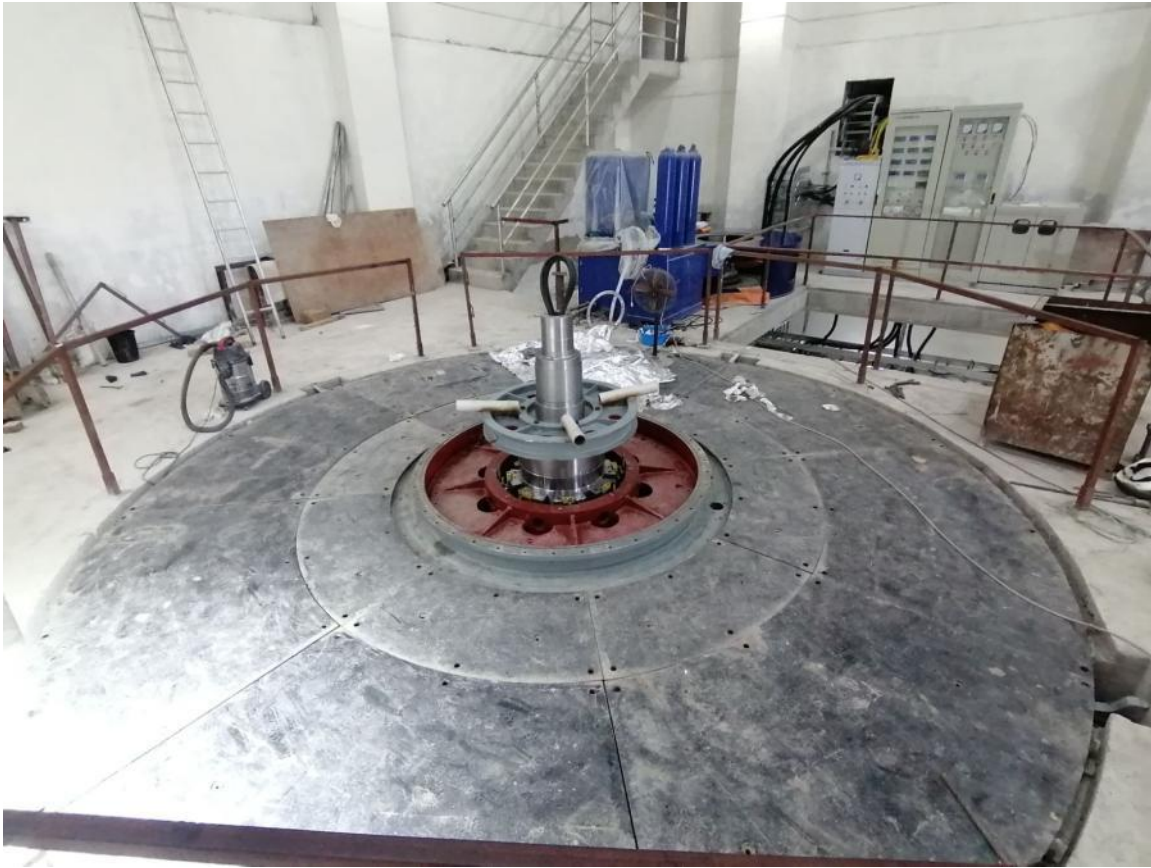
Figure 10: Top cover installation at machine unit 1
