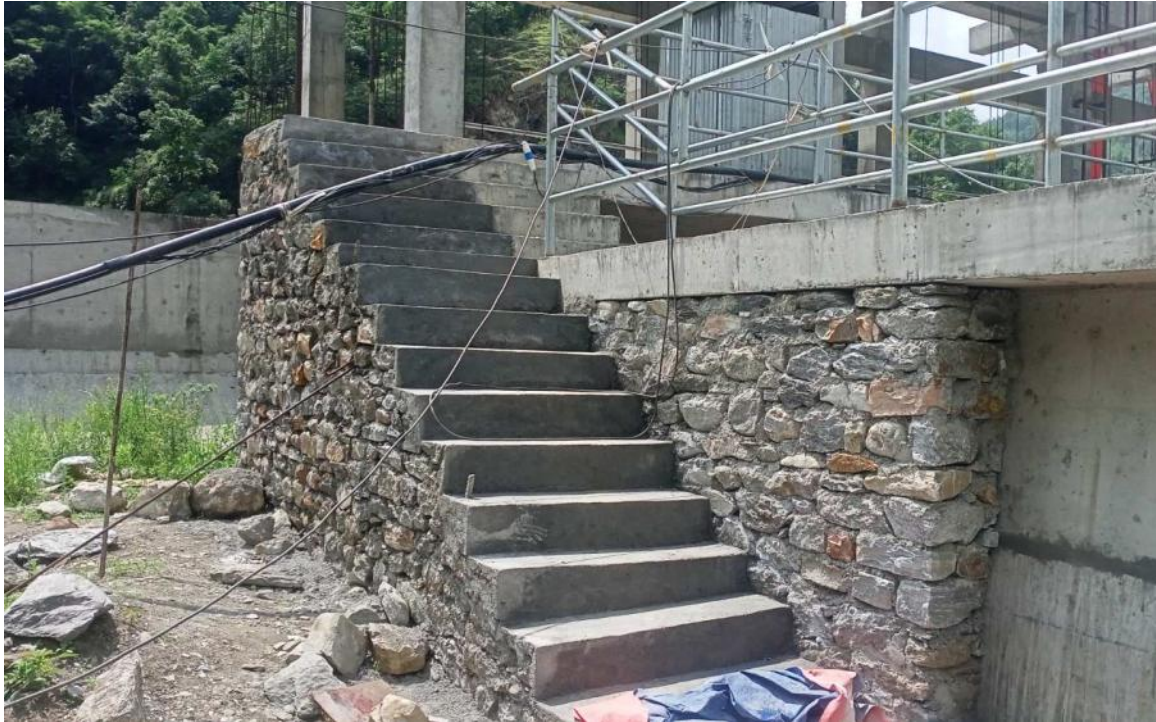
Figure 22: Stair for access to the intake gate operation platform
