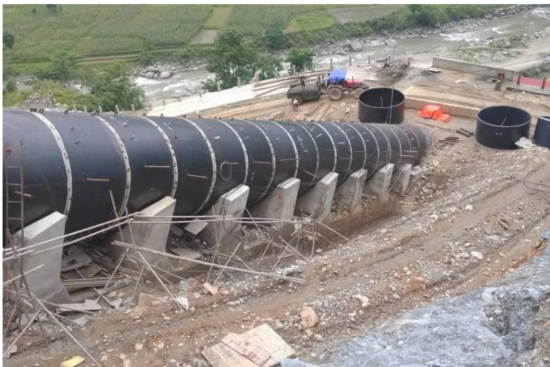
Figure 9: Pipe installation between anchor block VB01 and VB02 of penstock
