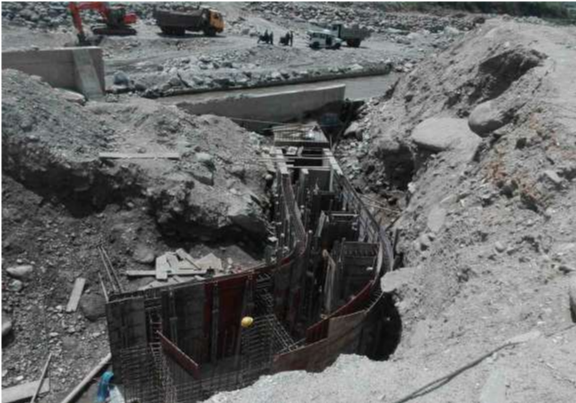
Figure 24: Construction of fish passage
