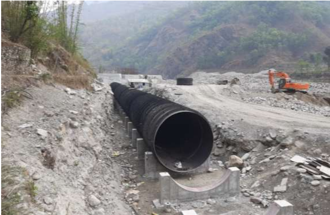
Figure 15: Headrace pipe from conveyance tank
