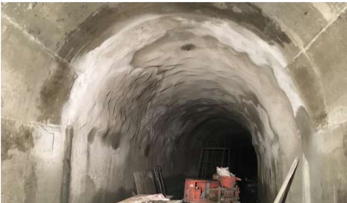
Figure 7: Junction between concrete lining and shotcrete-concrete section at Face 6
