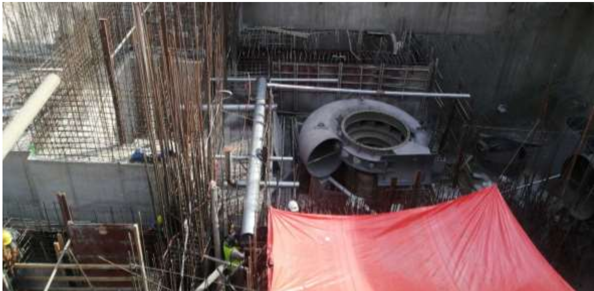
Figure 18: Pipeline layout in Bay 01
