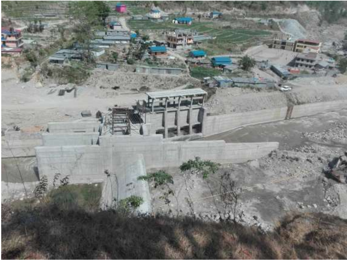
Figure 1: Weir, Intake and Undersluice from top
