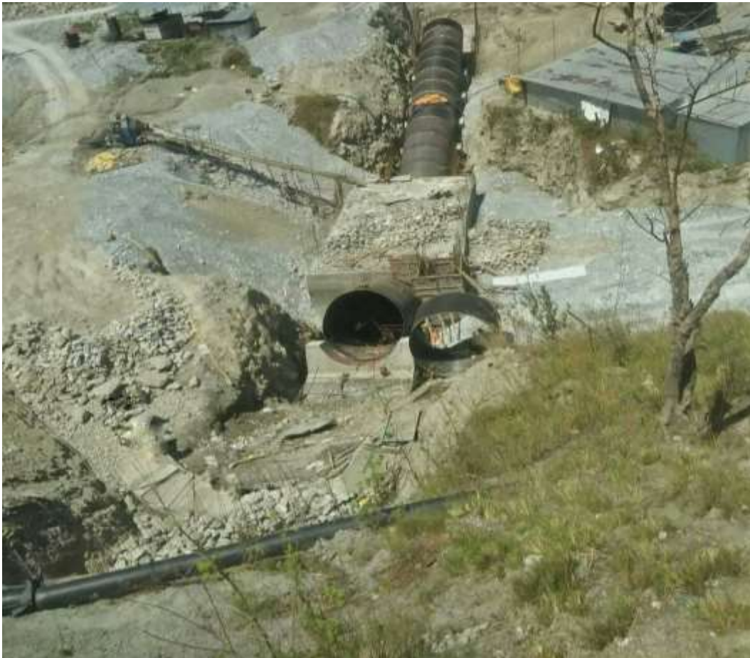
Figure 22: Irrigation canal across the siphon crossing for public use (concrete slab)
