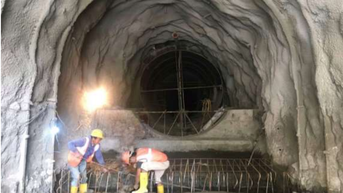
Figure 6: Construction of saddles at Poku Outlet portal
