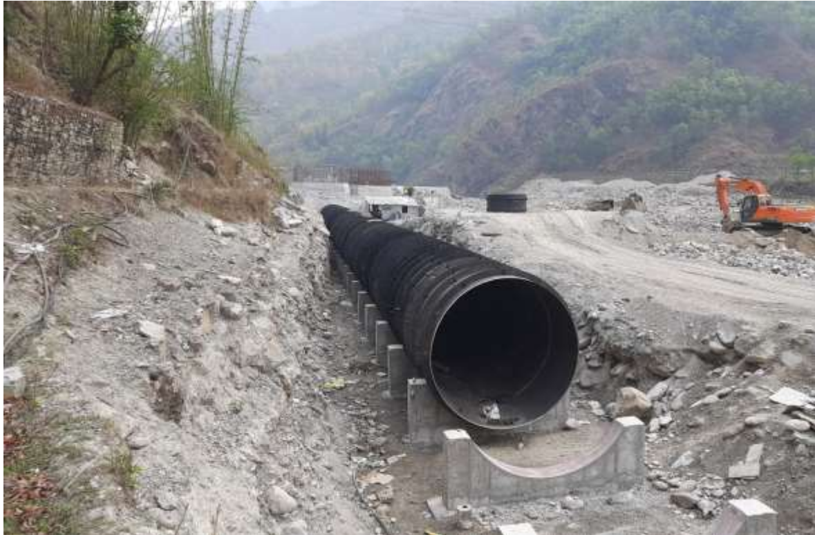
Figure 4: Headrace pipe and saddle support
