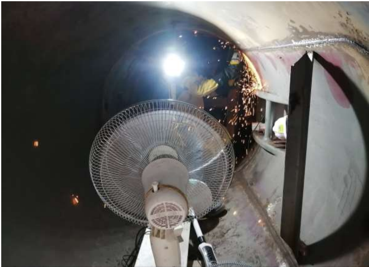
Figure 33: Welding of spiral case from inside
