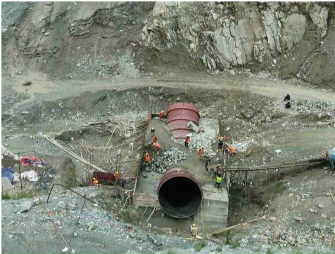
Figure 26: Plum concrete at Poku crossing
