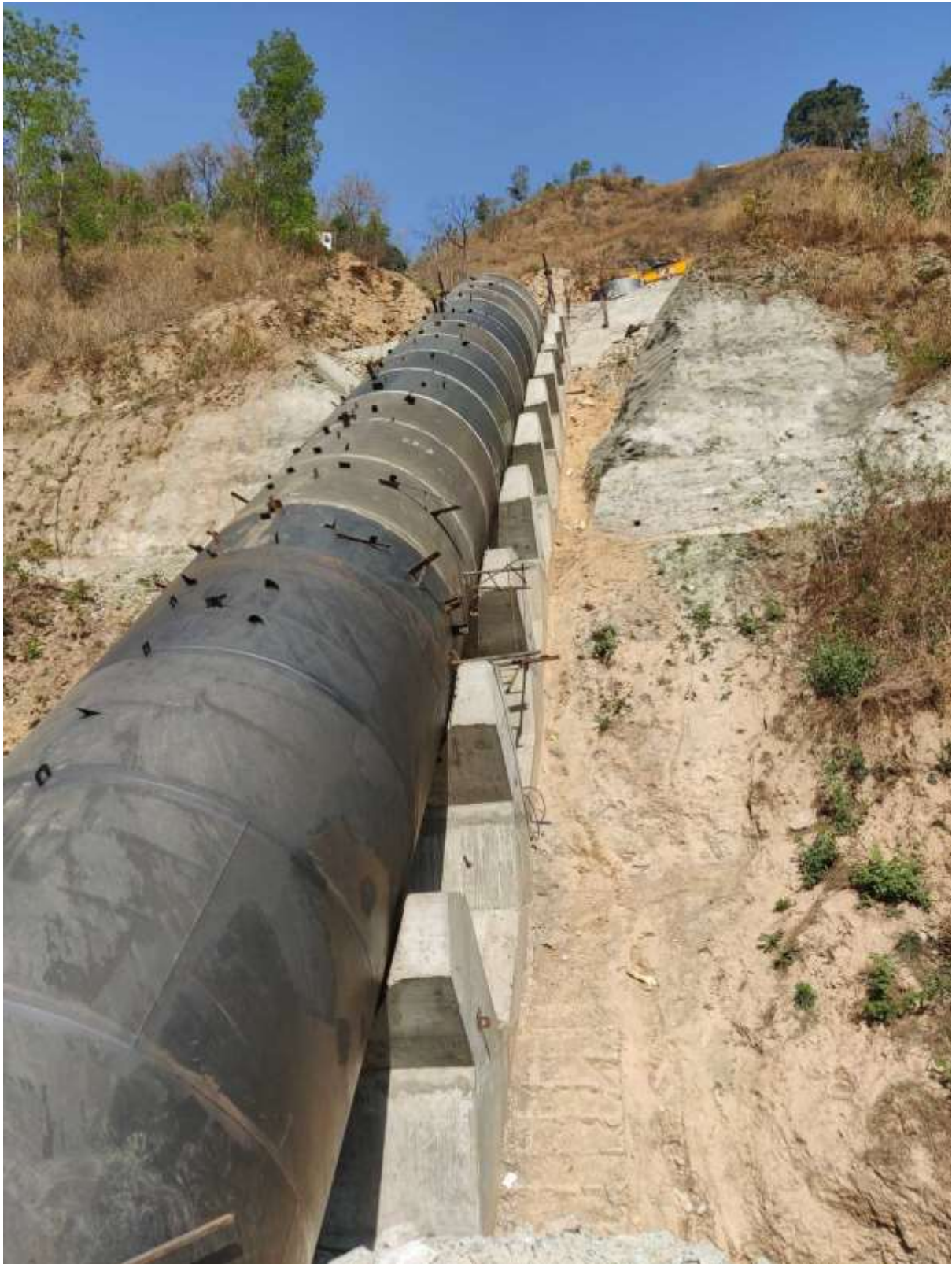
Figure 17: Penstock pipe alignment between wyee and VB02
