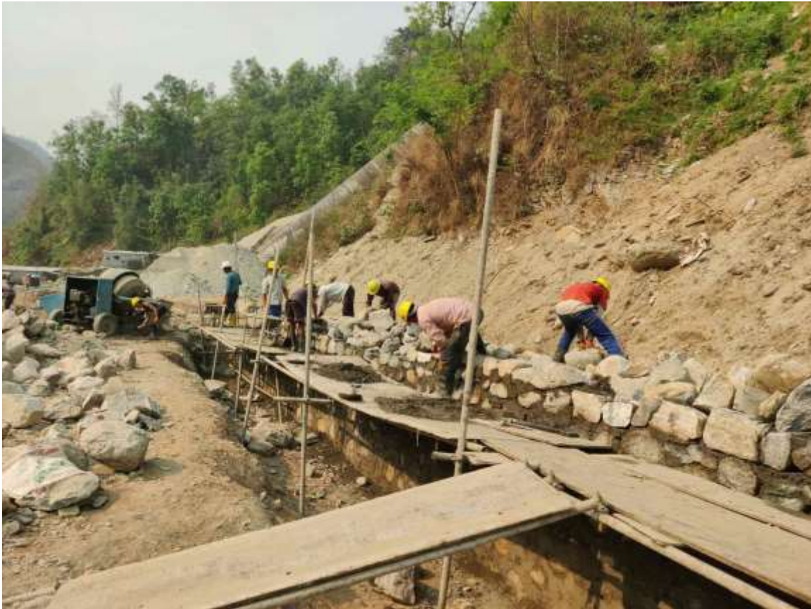
Figure 29: Stone masonry works for switchyard protection
