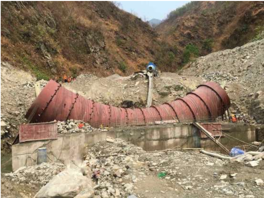
Figure 10: Pipe at Poku crossing anchor block
