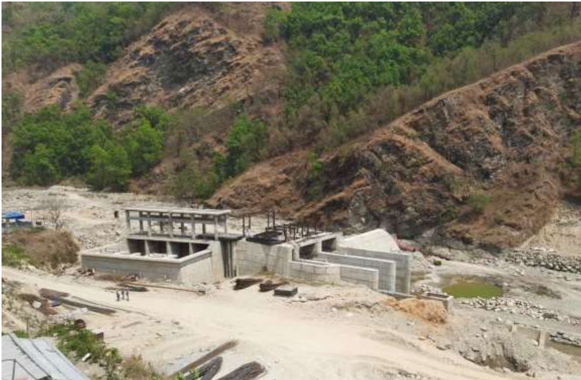
Figure 23: View of weir, intake and undersluice
