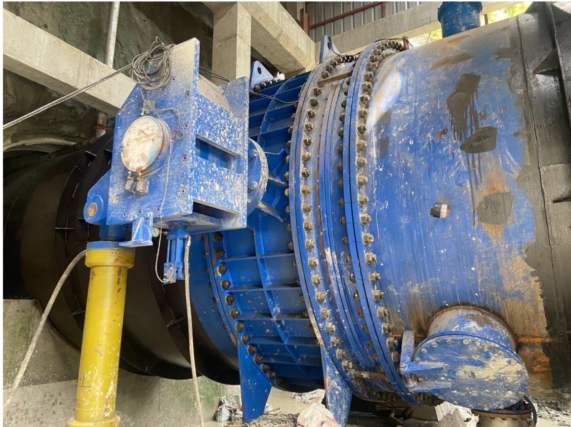
Figure 19: Penstock protection valve
