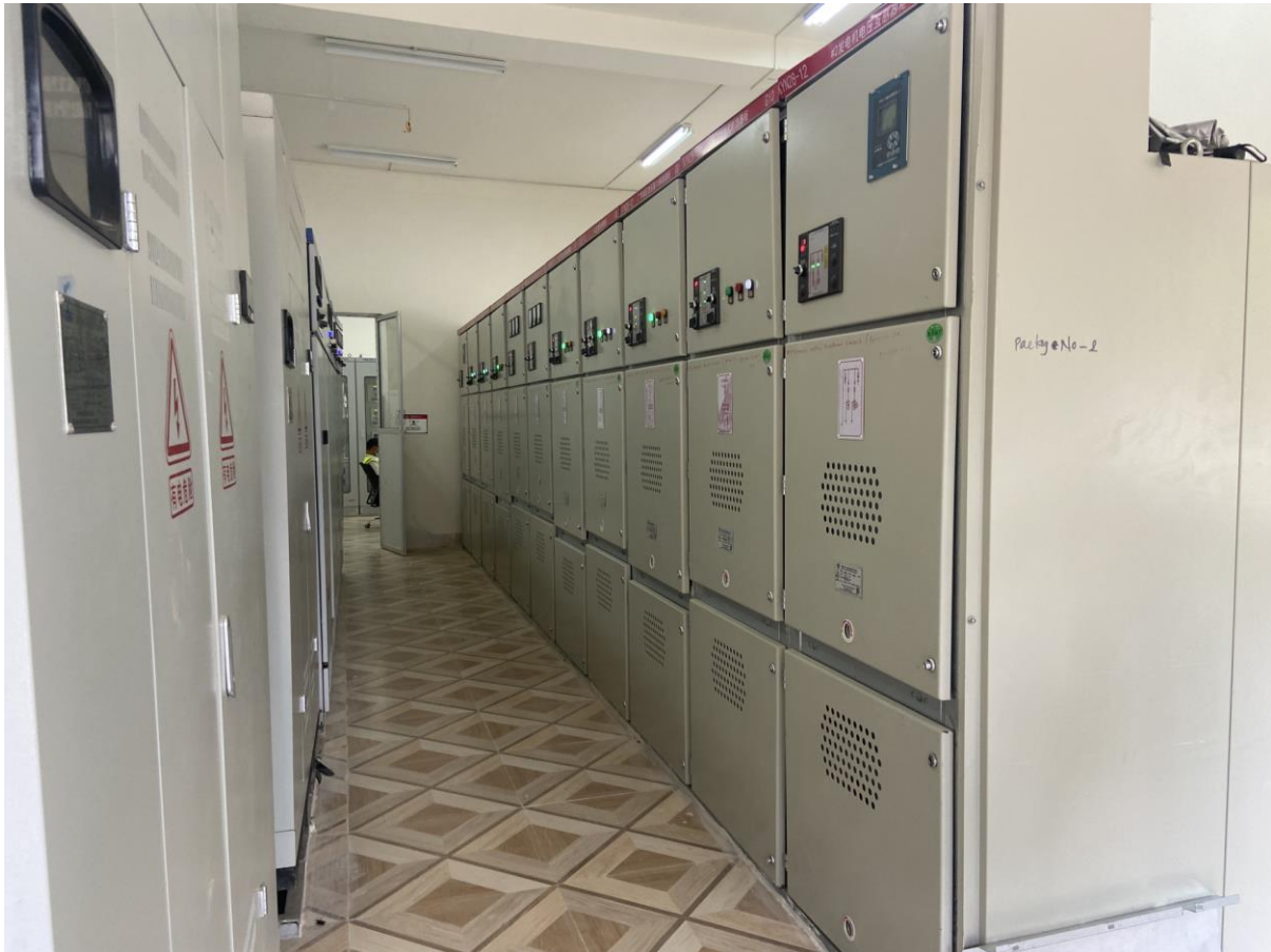
Figure 16: High and low voltage Cubicle room
