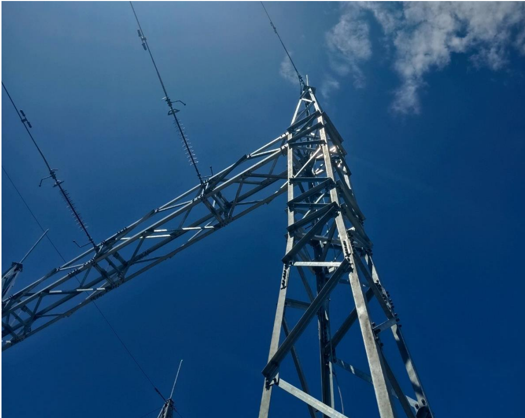
Figure 20: OPGW stringing between gantries at New Khimti Substation
