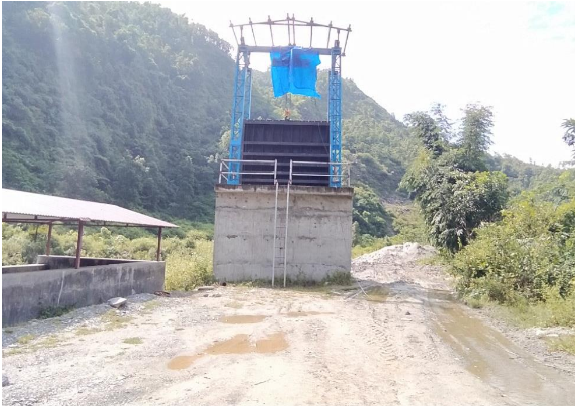
Figure 14: Installation of tailrace stoplog
