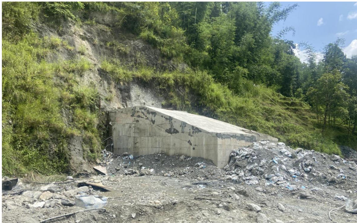
Figure 4: Seti outlet portal anchor block
