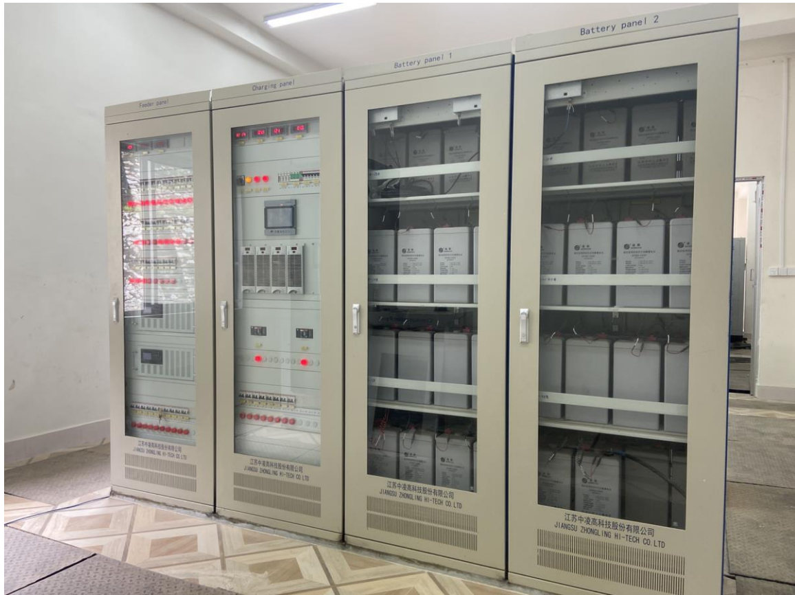
Figure 31: Feeder panel, charging panel and battery panels at the control room
