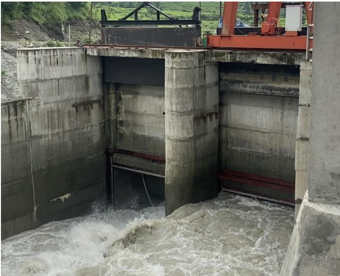
Figure 26: Undersluice stoplog
