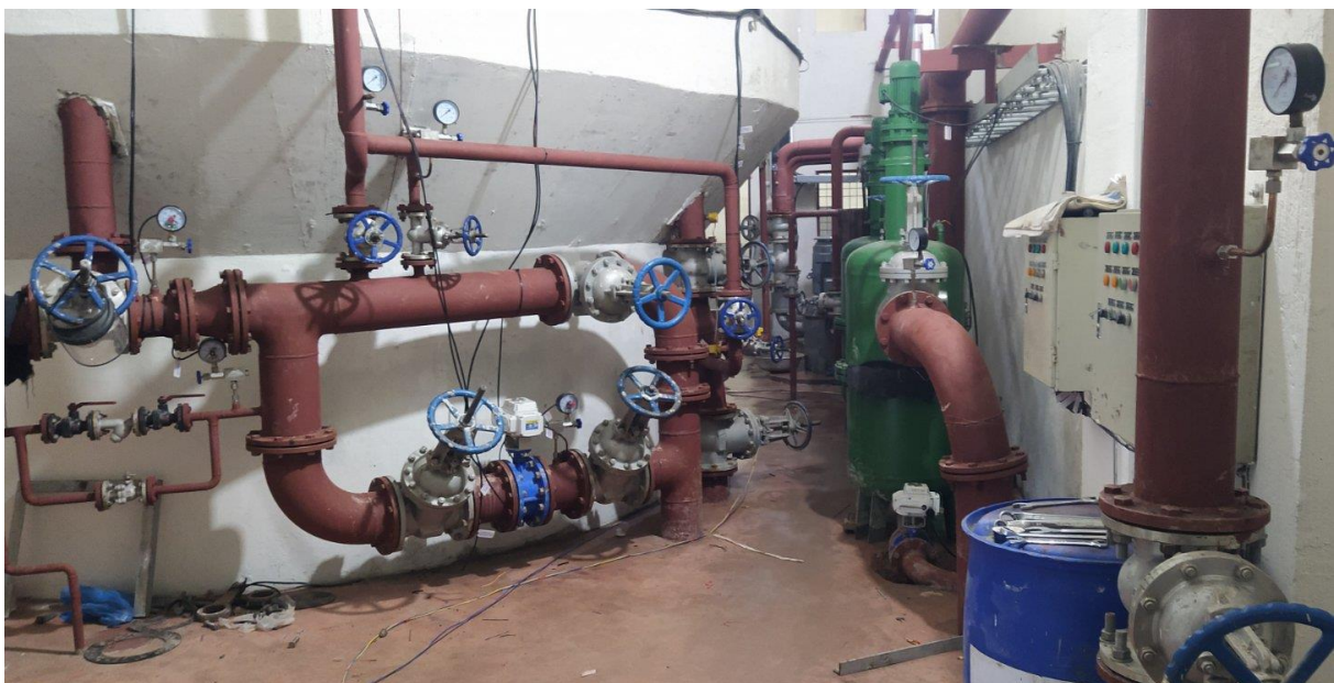
Figure 17: Cooling pipeline system in the powerhouse
