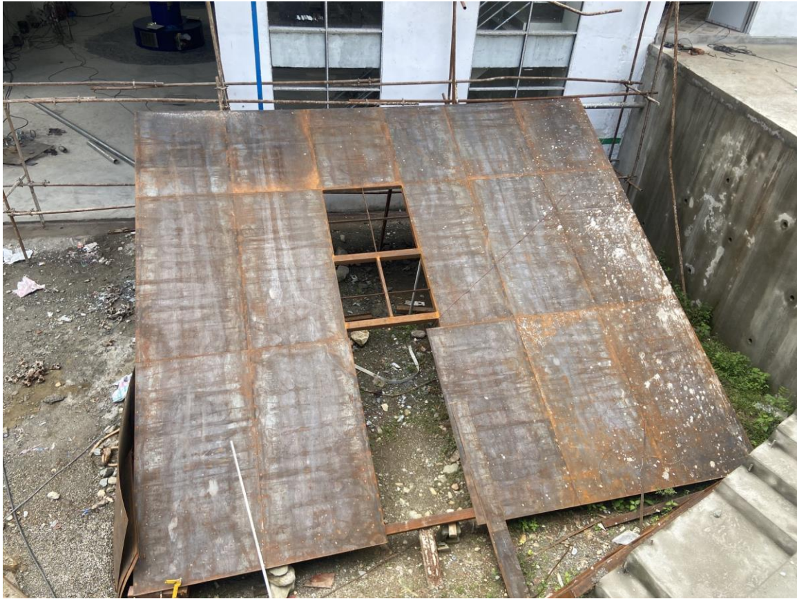
Figure 29: Fabrication of the powerhouse main door
