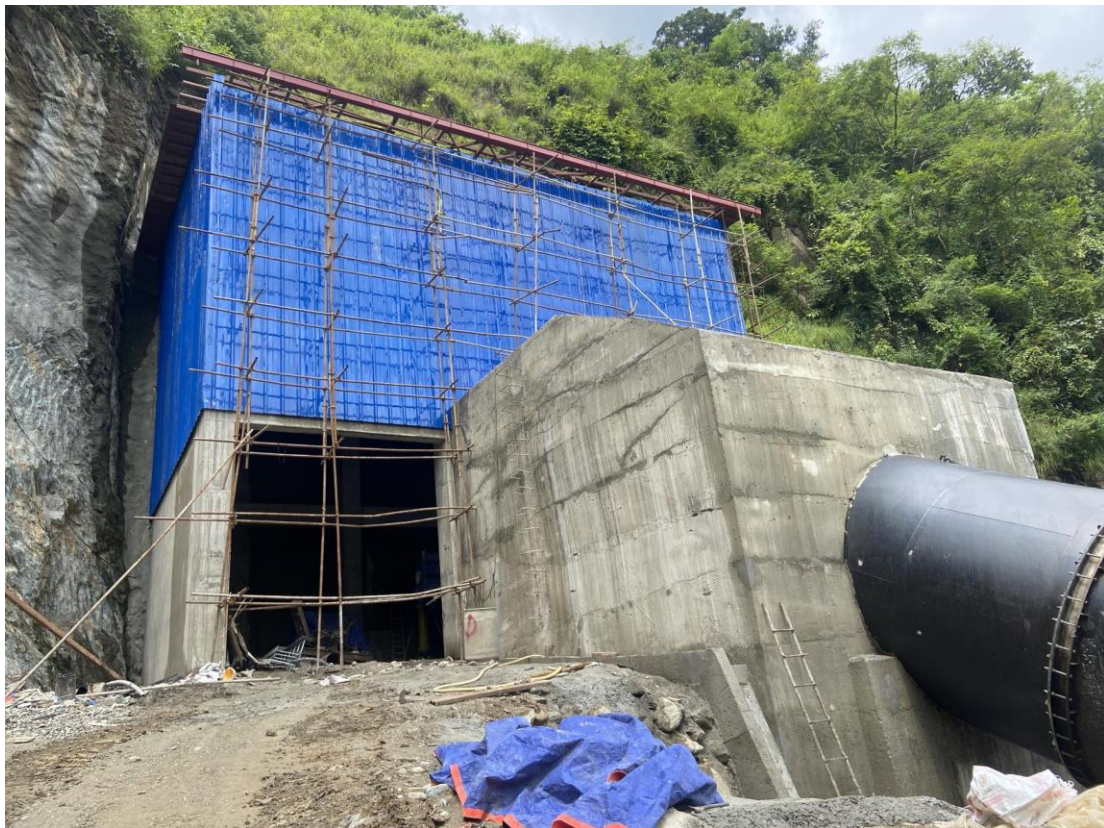
Figure 9: PPV house and penstock anchor block VB01
